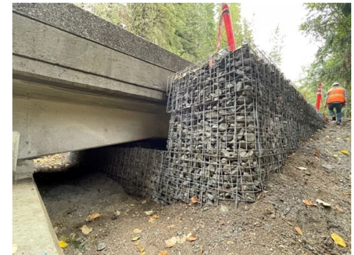
Looking Under the Finney Creek Bridge
